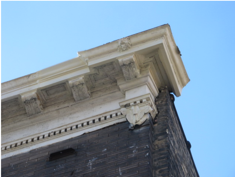
Upper Cornice – West End – repaired with formed sheet metal
