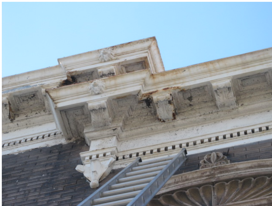
Upper Cornice – rusted holes in metal
