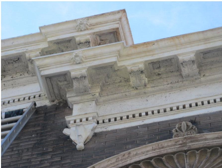
Upper Cornice – repaired with formed sheet metal
