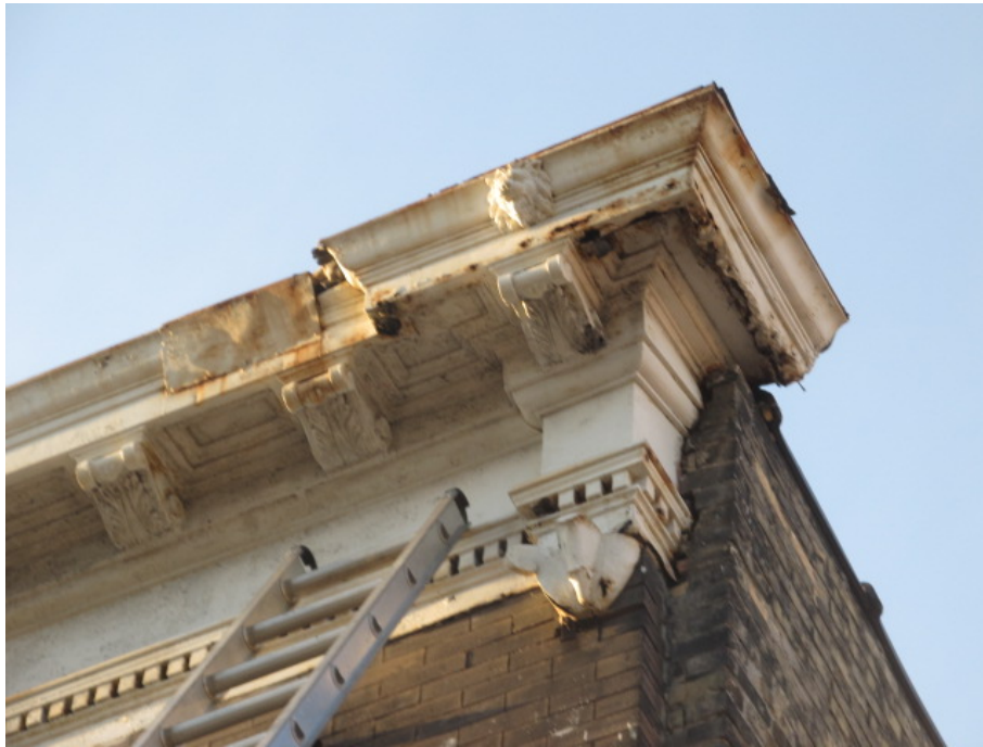
Upper Cornice – West End - improper repair - rusted holes in metal
