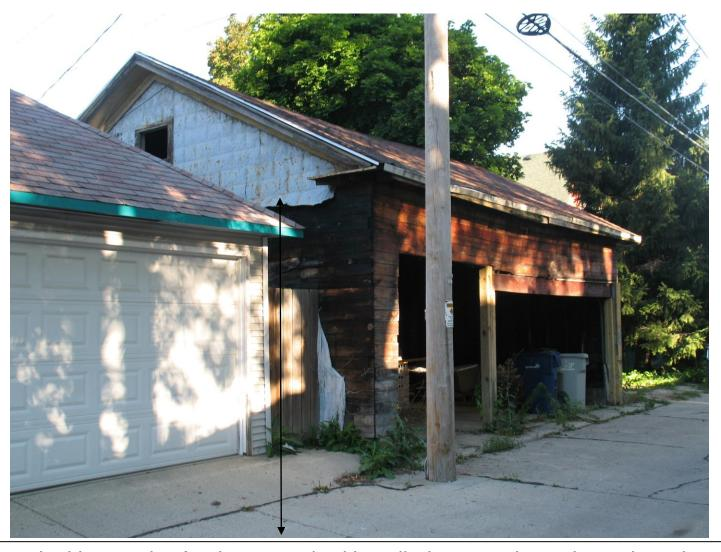
Rear garage looking north. A prior owner had installed stamped metal panels to the exterior. A number of the panels had been removed and no match could be found for them. The garage will get clapboard sheathing or carside sheathing.
