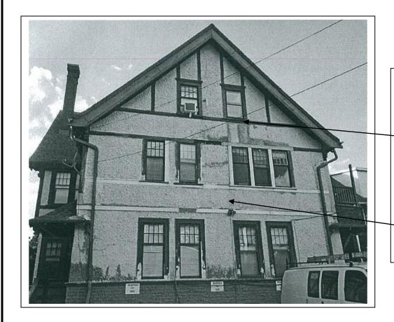
Stucco and wood trim are being repaired/replaced. Stucco repairs should have final texture to match original.
