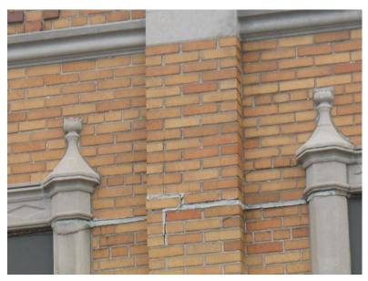
Horizontal fault lines will be cleaned out and anchored to inner wall and new mortar will be applied. The goal is to straighten the buckled piers or at least stabilize them. The steel lintels will be examined for possible repair and depending on the damage stone trim might be temporarily removed for access to the lintels.
