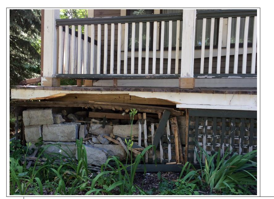
Close-up of damage. Damaged concrete blocks will be removed and new footings poured. Trim and lattice skirting will be replaced.
