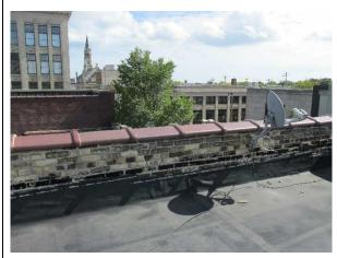
The south façade shows movement of the bricks away from the building, past repairs, and damaged mortar joints.
