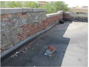
The photo below shows the gap where the building is seperating (west wall).
