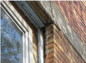
It appears that stone was added to the first floor at some point in the past as it does not appear original to the building. This stone façade shows cracking and sever outward bowing. Past mortar repairs also show cracking.
