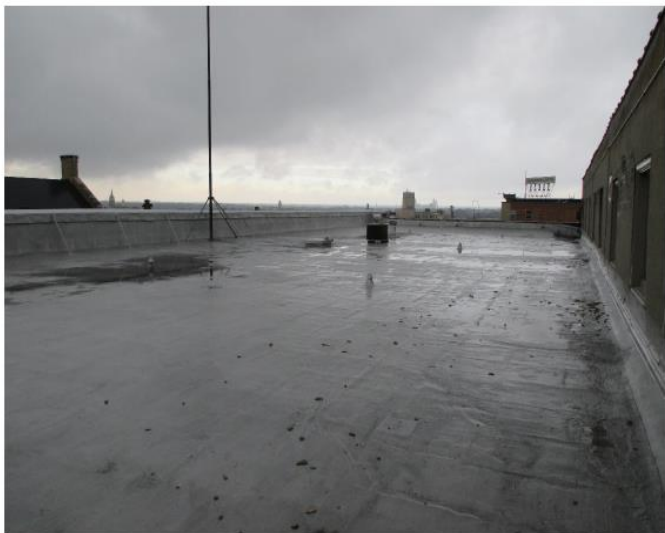
Photo 6 - 12.23.14: Main building roof looking southwest.
