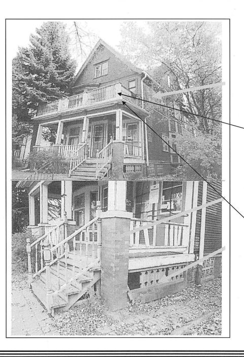
Note: upper and lower balusters do not match and are inappropriate for the house.
