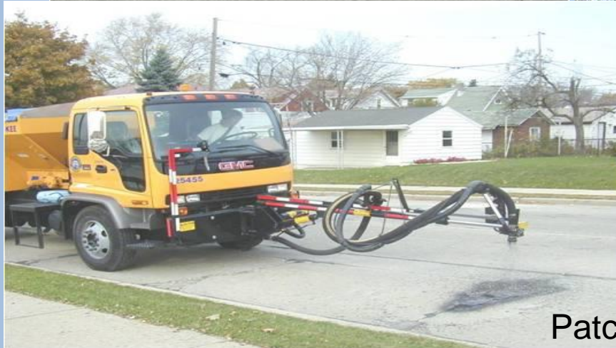
Crack Filling
