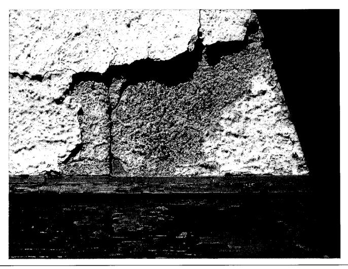
Stucco repairs were required at different sections of the house. At these sections the loose and cracked stucco will be removed, new lath will be applied and a base and scratch coat applied. Flaking paint on wood trim and sound stucco will be removed and surfaces prepared for new final coat of stucco and paint on the wood trim.
