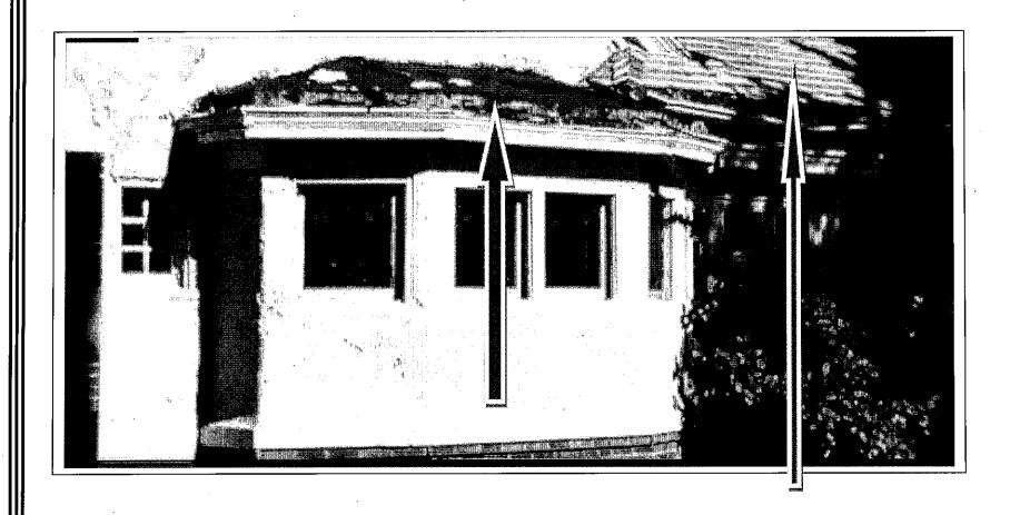
Roof on south bay is deteriorated. Built in gutters to be rebuilt with copper. Gutters next to bay are deteriorated. Make sure compatible metals to be used to prevent corrosion.
