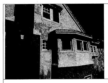
South bay roof structure requires repair, rebuild and resheathing with metal or copper. Rebuild built-in gutters. Preserve roof details here.
