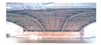
The leaf is raised and lowered by moving the large segmental racks mounted beneath the girders.
