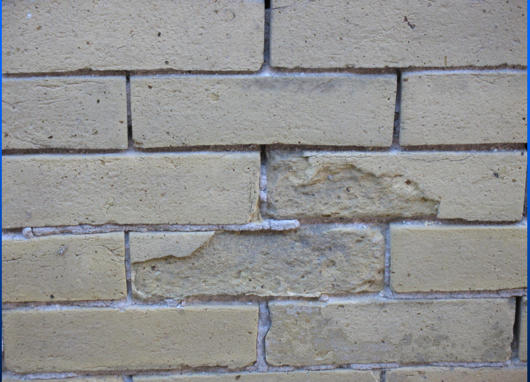
Brick damaged from hard mortar
