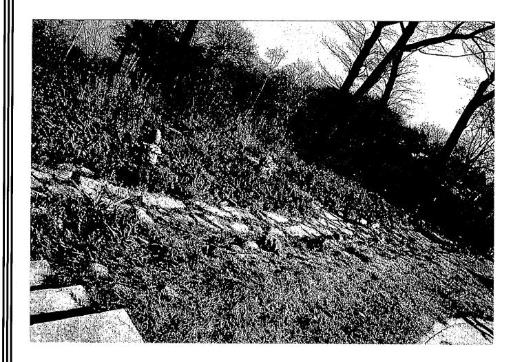
Limestone step treads and flagstone switchback paths will be repaired and reset down bluff
