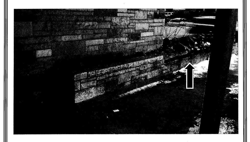
Lannon stone clad planter is original to the building's design. River rock replaced plantings c. 1970s. Vandalism has resulted in loss of stone veneer.
