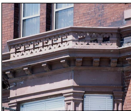
Sheet metal balustrade atop the bay
