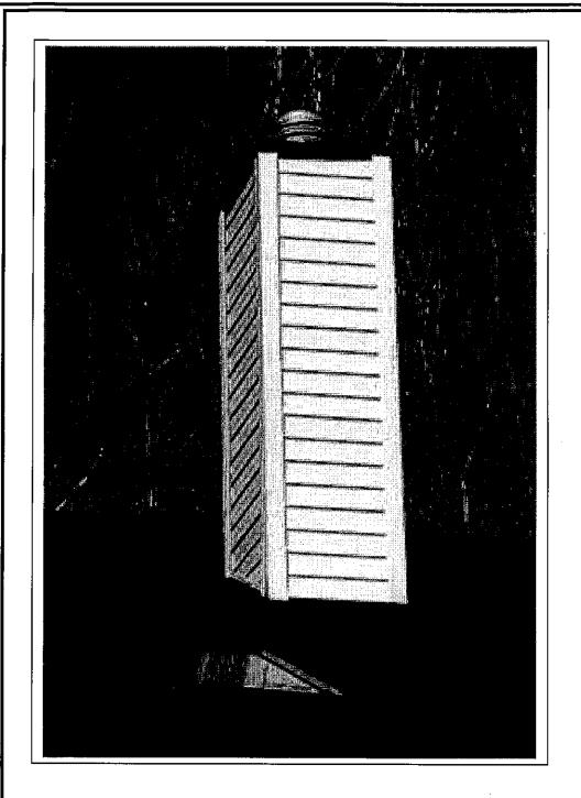
A chase such as this and chimney top will be installed around the bare metal pipe that will be installed by Fire Place LLTD. A separate contractor will be constructing the chase.
