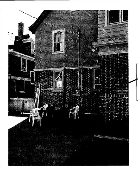
Install new split system a/c unit on grade, next to foundation in back of house. Run line set up to second floor. Ideally line set should be on an inside corner to minimize its appearance.
