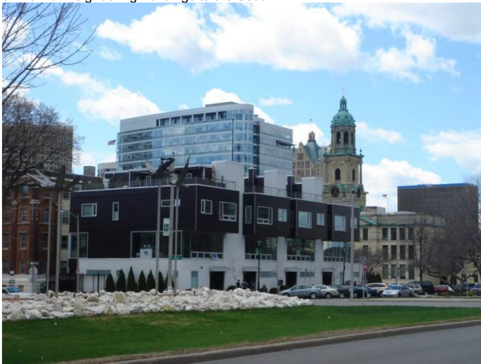
6. View of Neighboring Buildings to the South
