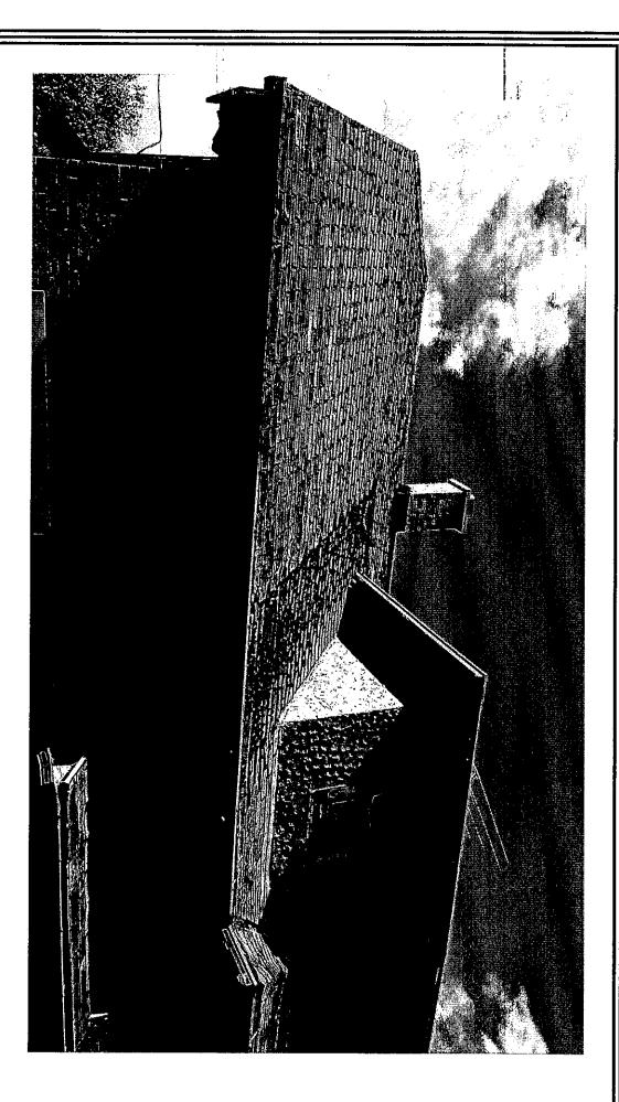
Rear chimney to be retained and tuck-pointed if necessary. Chimney can be capped so as to maintain the existing appearance from ground level. Stucco on dormers must remain undisturbed. New K-style gutters to be isntalled on flat fascia boards.
