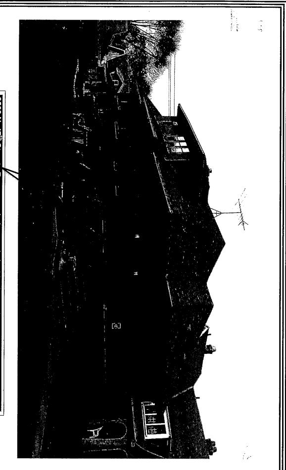
2563 N. 47<sup>th</sup> Street. Remove existing asphalt shingles and gutters. Install new GAF Timberline Natural Shadow Shingles in either Bark wood or Hickory color. All dormers chimneys and other architectural details must remain undisturbed
