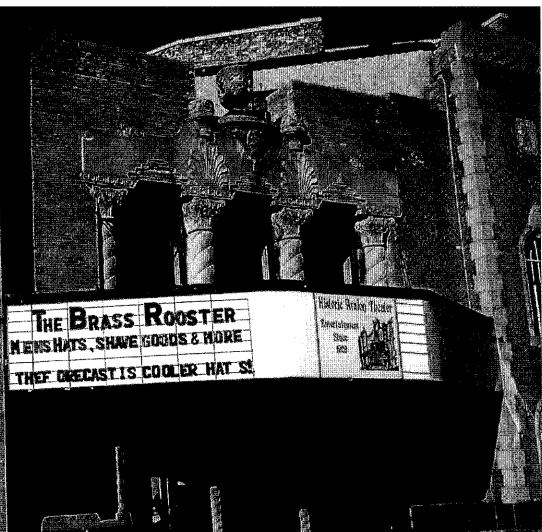
Only the central part of the theater will be restored at this point. Original steel sash (five in total), will be restored. Old doors will be removed and replaced with new matching doors using the historic pulls. A new sign will be installed, but that will be done on under a separate COA
