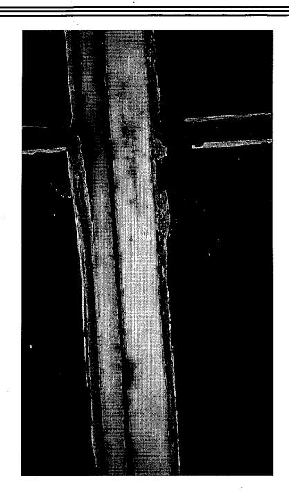
Where existing steel sash are severely damaged, the old piece will be remove and a new match steel piece will be welded in place.
