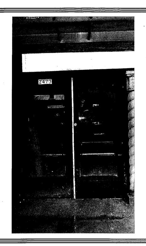
Original door pulls will be salvaged and re-installed in the new entry doors which will be made to fit the existing openings. Three sets of the doors, because of their narrow overall width will have to be made with a fixed sash alongside the standard entry door.
