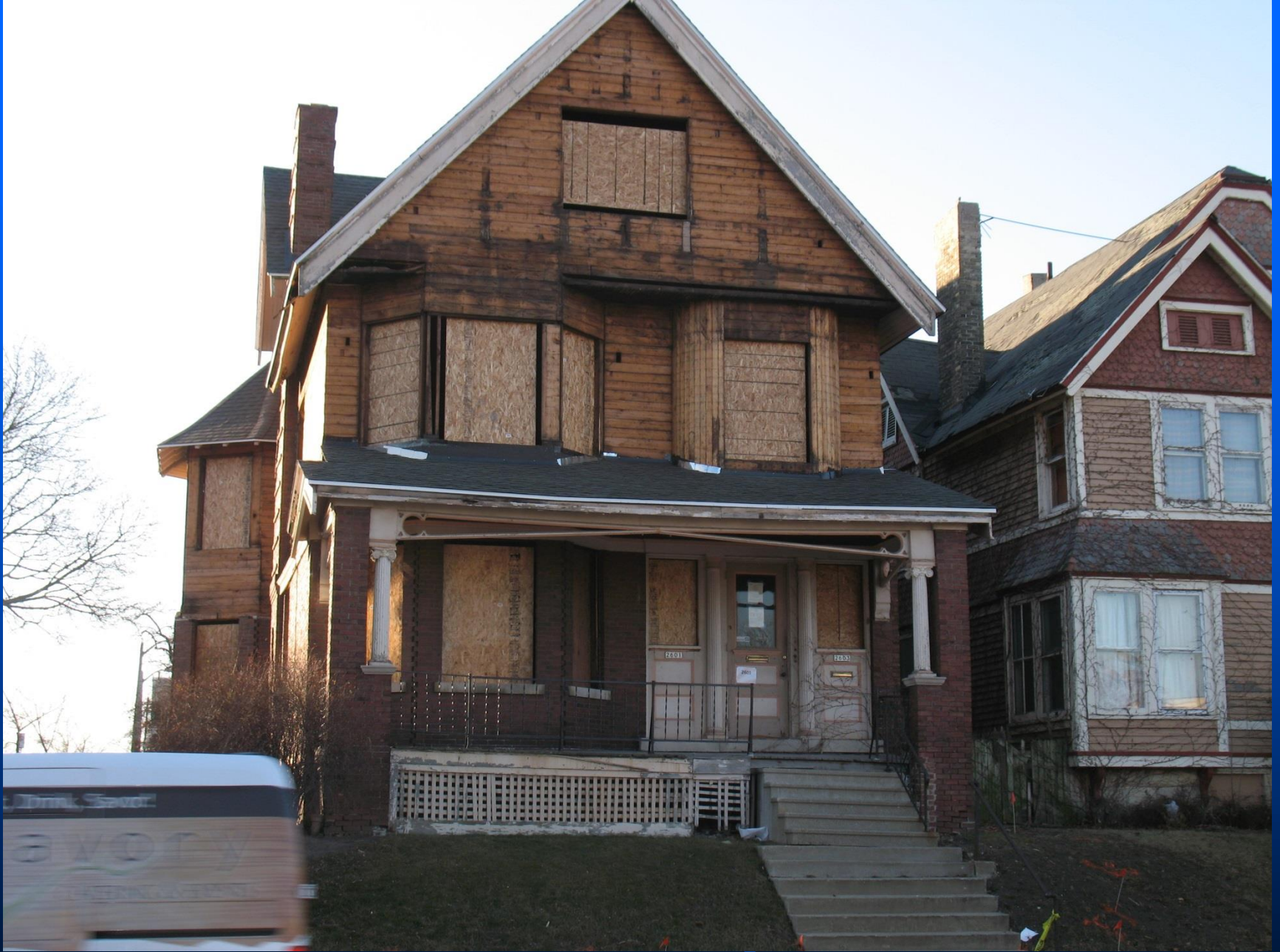
2601 WEST WELLS STREET STRIPPED AND AWAITING VINYL SIDING
