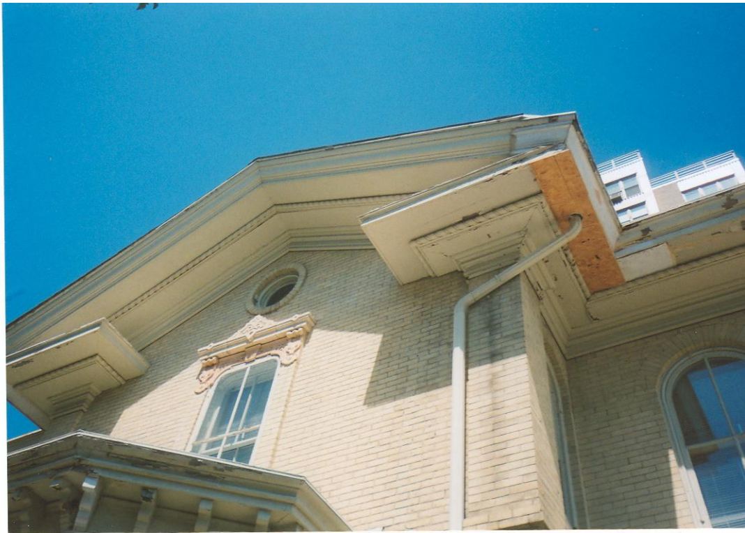
Soffit damage at the Peck House
