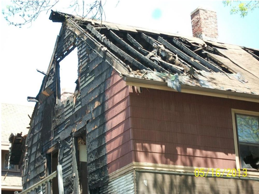
The fire-damaged duplex had been clad in cement asbestos siding.
