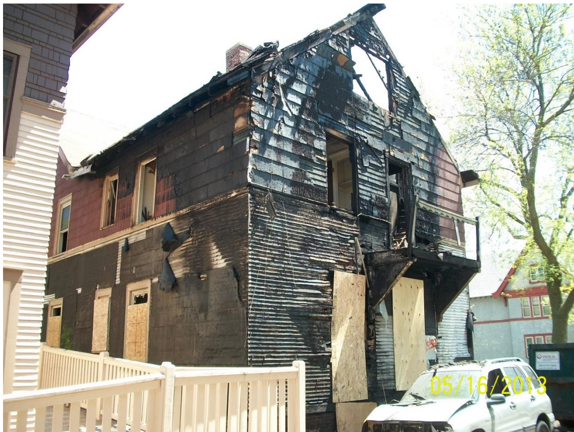
The fire-damaged duplex had been clad in cement asbestos siding.
