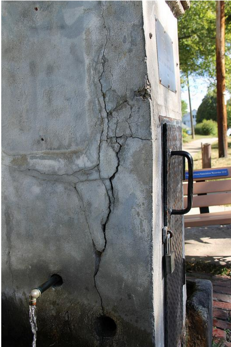
Cracks on wellhead before restoration
