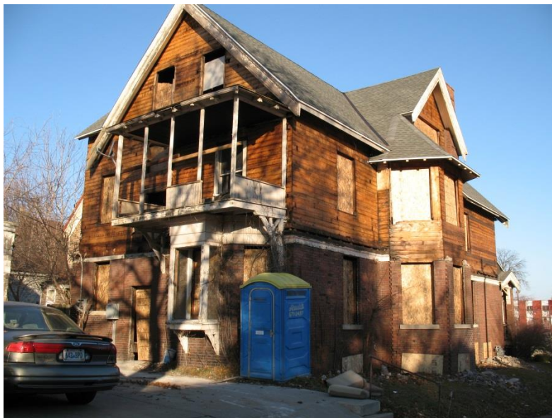
2601 West Wells Street stripped of its original ornamental shingling in preparation for vinyl siding.
