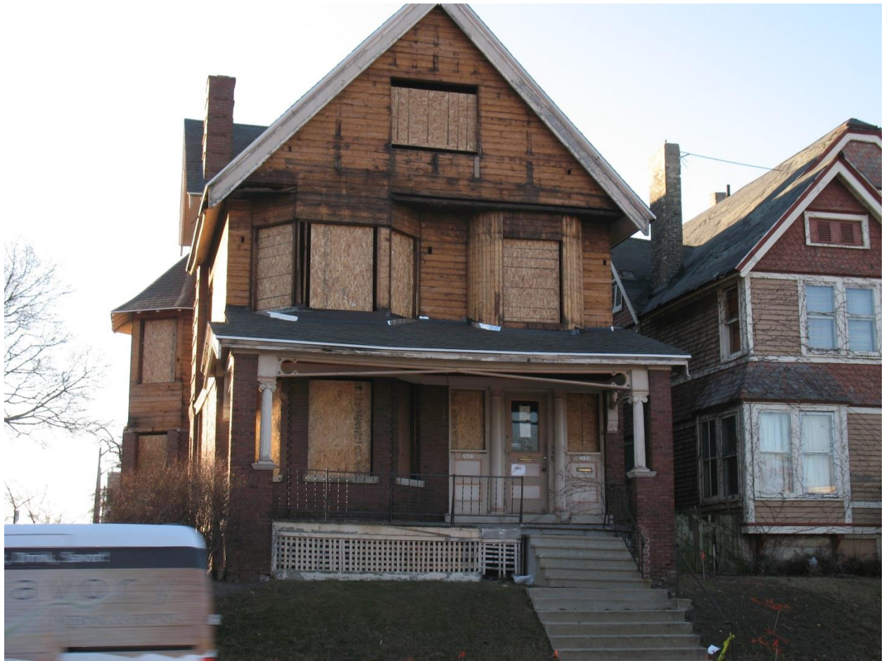
2601 West Wells Street stripped of its original ornamental shingling in preparation for vinyl siding.
