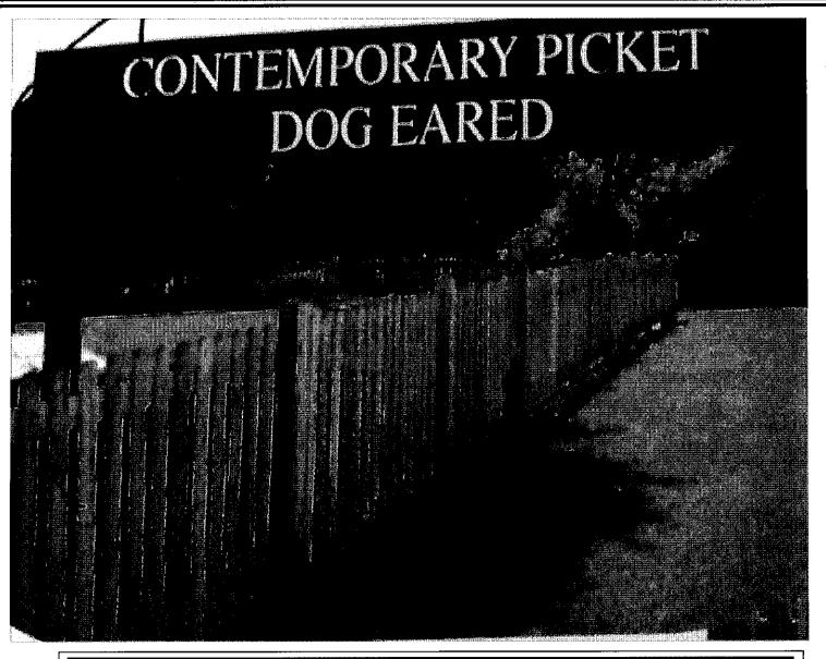
Dog-ear style wood picket fence, 4 feet in height, to be installed in rear yard between garage and house. "Good side" to face neighbor. Fence must be painted or stained upon completion.
