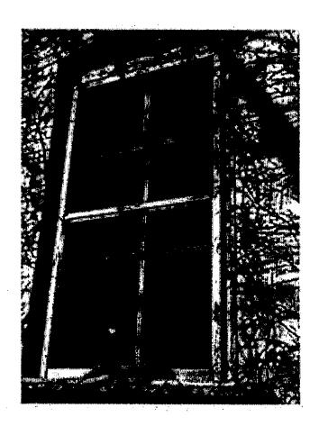
Typical existing aluminum storm on rear house (shown) that will be replaced with a new all-wood storm both inside and out. New storms will match the meeting rails of the prime windows behind it.
