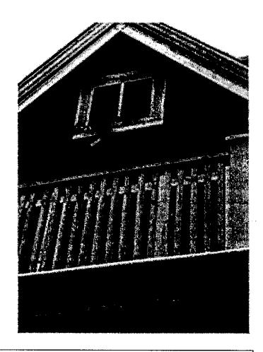
Replace sidewall shingles in gables on front house as need with matching, new, clear shingles.
