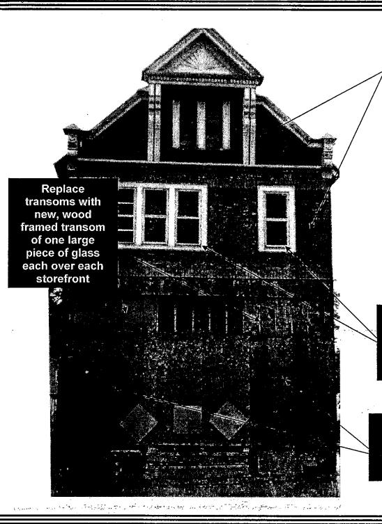
Remove all asphalt siding on all sides of the building restore original wood siding and wood shingling underneath or replace with new, clear wood to match original as needed. All wood
