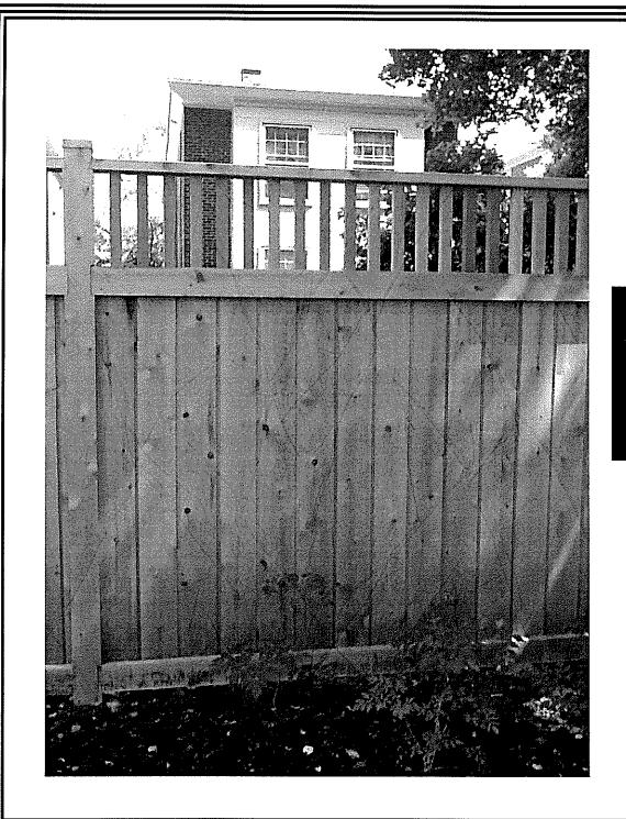
Design of wood privacy fence to be installed south of driveway. Fence will match existing wood treillage fence in design and
