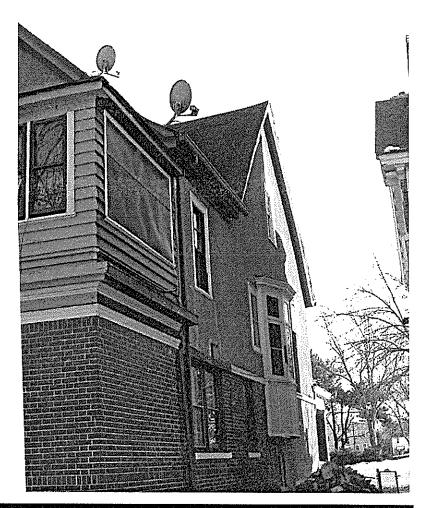
Tuckpoint brick where needed, but only loose or missing mortar should be replaced. New mortar must match the original in terms of color, texture, hardness, joint width and joint finish.
