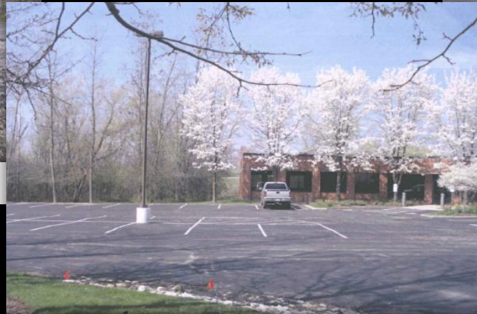
East face and south end of building. Photo taken from the southeast edge of the parking lot.
