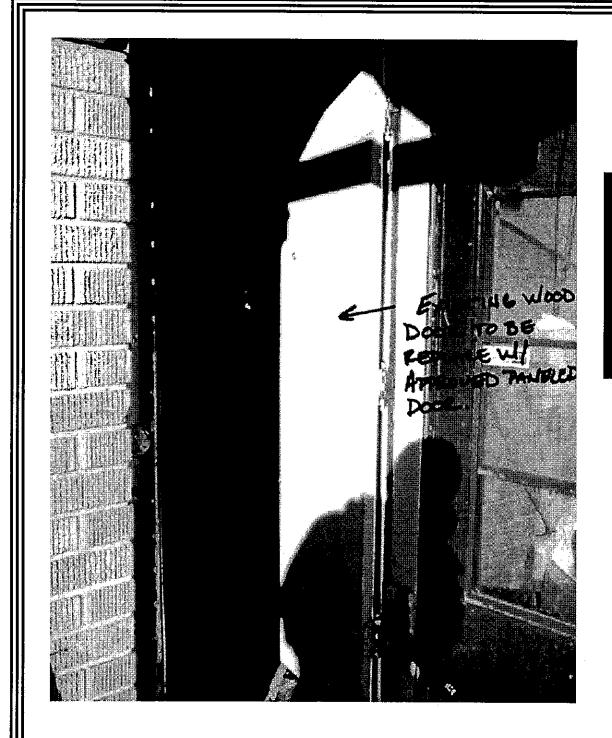
Rear Elevation. Four panel wood door to be installed in place of existing flush door and a full-view wood storm installed over that. All wood must be painted upon completion
