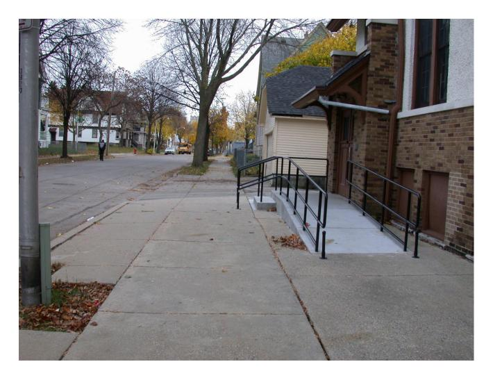
CCF 110494 2176 North 39<sup>th</sup> Street 11-11-2011 Looking east at platform, ramp, step and railing in south sidewalk area of West Garfield Avenue. There is 5 feet clearance for pedestrian traffic adjacent to the railing and step.
