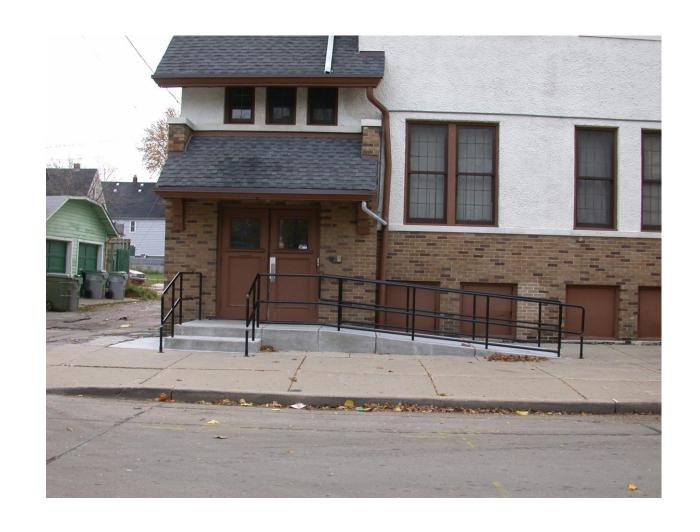
CCF 110494 2176 North 39<sup>th</sup> Street 11-11-2011 Looking south across West Garfield Avenue at barrier free access ramp, platform, step and handrails.
