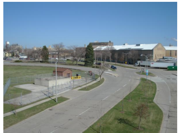
Overview of sub-area B-2, looking northwest
