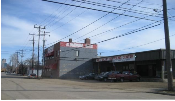
A recycling facility in District B, sub-area B1
