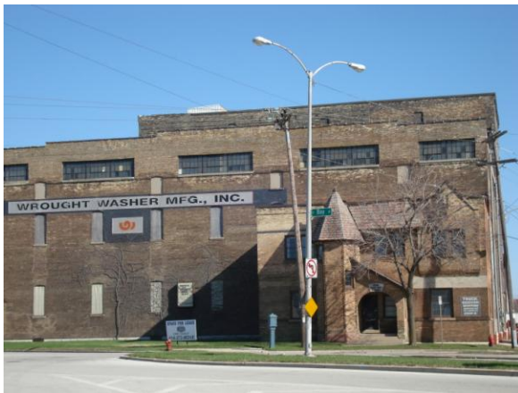
Wrought Washer, E. Bay St., sub-area B-2
