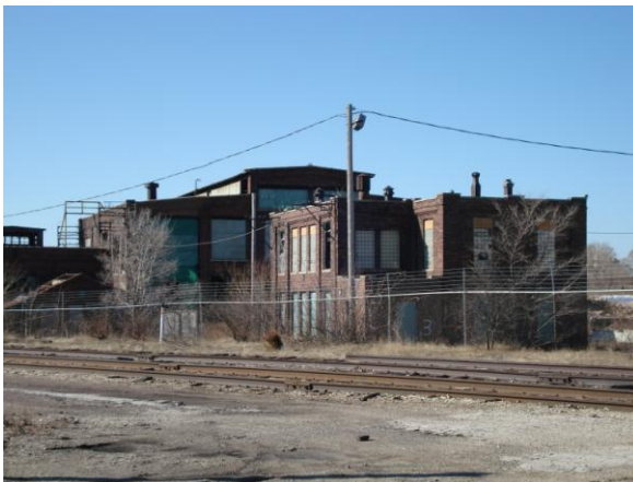
Vacant buildings at former Solvay Coke site, sub-area B1
