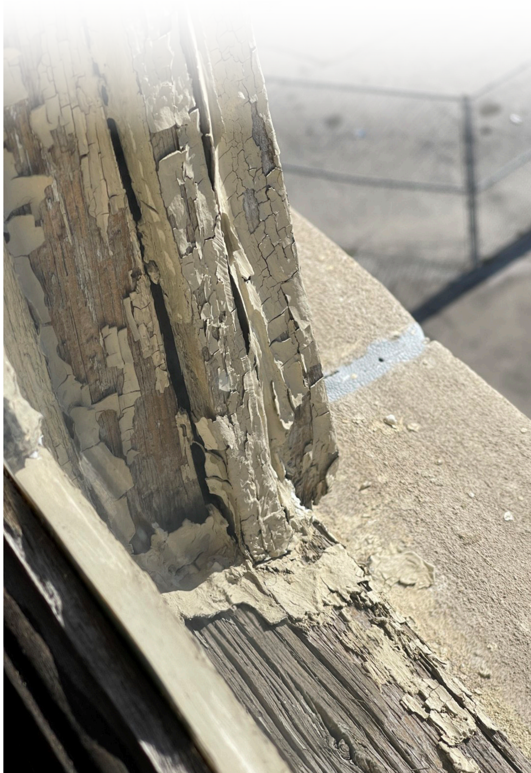
Existing window deterioration
