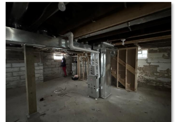
4369 N 26 th Street - Basement
