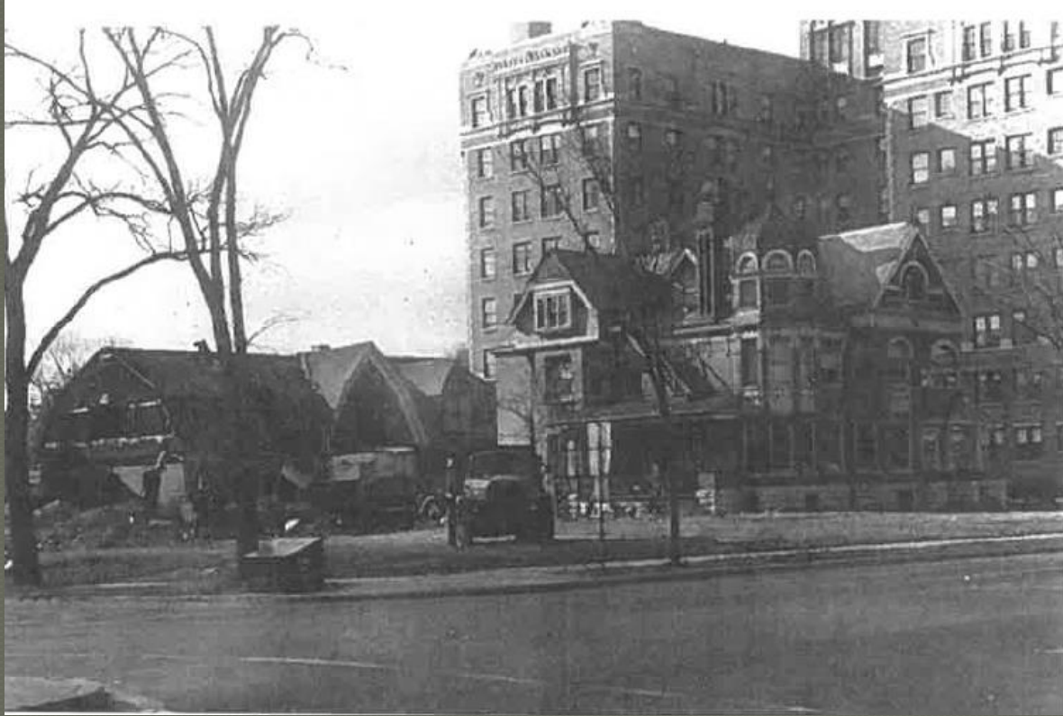
1957 – Millerand Apartment & Mayer House
