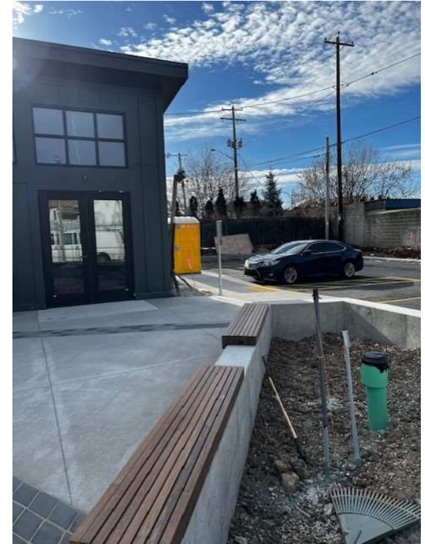
Concrete pavers and seating units
