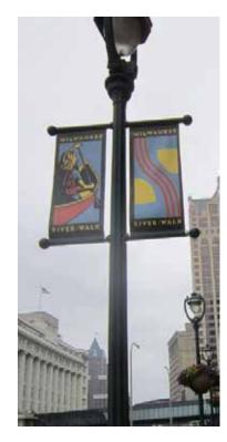
**EXISTING HARP LIGHT POLES** Remove existing finish, repaint and reinstall
