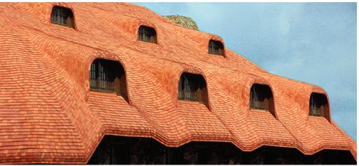
Ludowici's flat slab shingle tile has a smooth surface and square butt creating a clean look suitable to any architectural style. Flat slab tiles are available in  $\frac{3}{8}$ " and  $\frac{5}{8}$ " thicknesses and standard and custom matte colors, mists and blends. See the *Colors of Ludowici* brochure for more information about our extensive color program.
