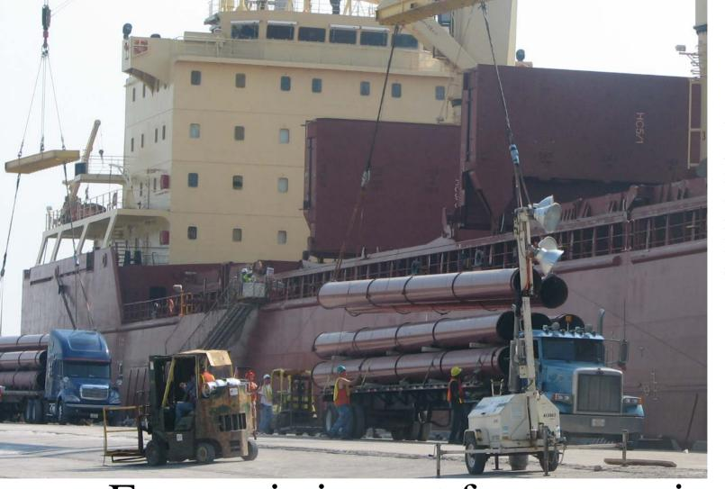
3 lifts per truck Average 20 minutes to load one truck; four trucks loaded simultaneously.
