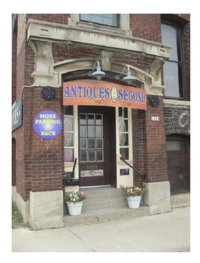
CCF 101217 224 W Washington St 4-4-2011 Looking west at the sign projecting into the west sidewalk area of S 2<sup>nd</sup> St. At 8 feet 6 inches above the sidewalk grade, there is less than the 10 feet of clearance required by Section 244-10 of the Milwaukee Code of Ordinances.
