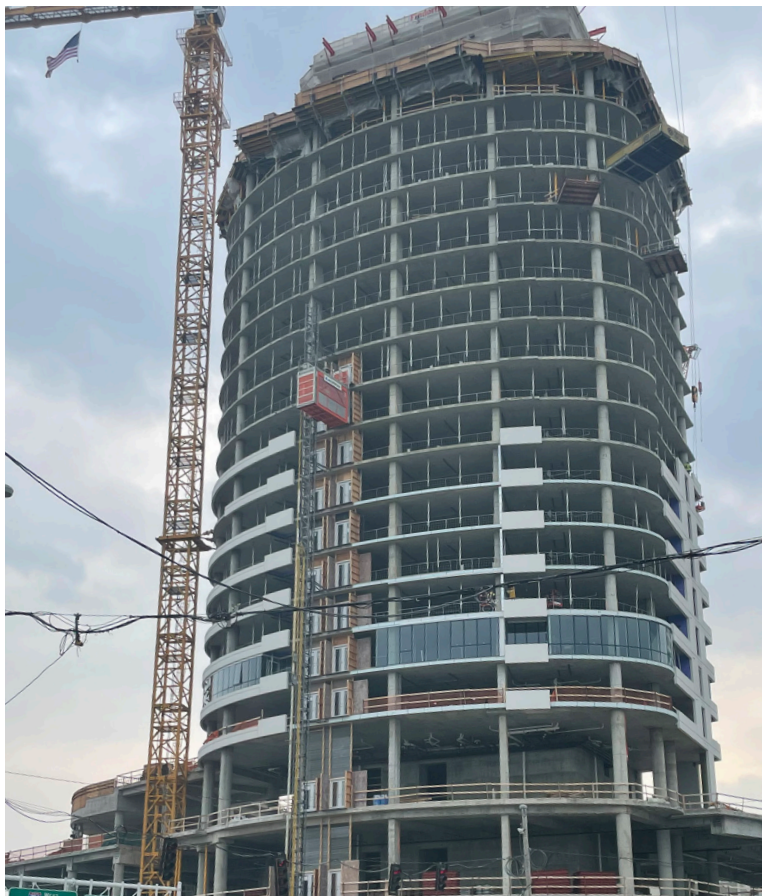
Work Progressing Summer 2023.
