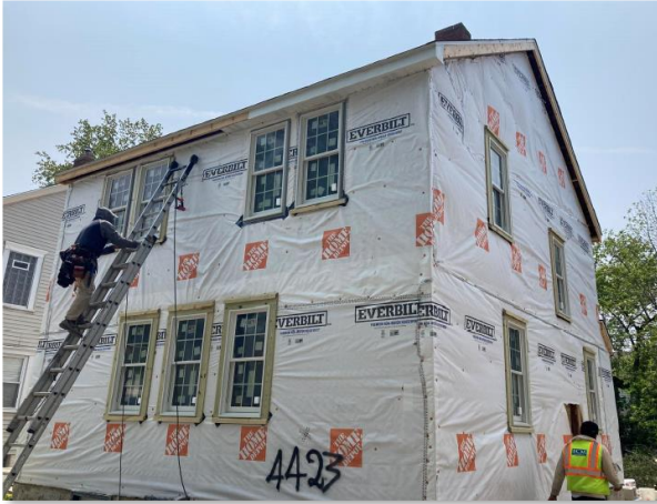
4423 N 25 th Street – Back Elevation
