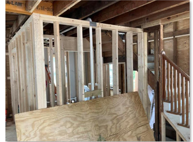
4423 N 25 th Street – Interior Framing
