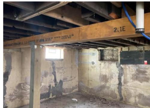
4423 N 25 th Street - Basement
