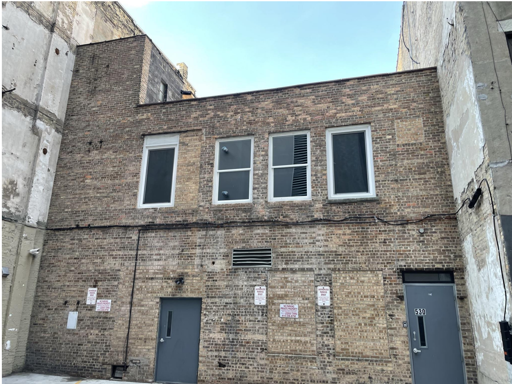
2023 photo of rear: the four second floor windows will be replaced
