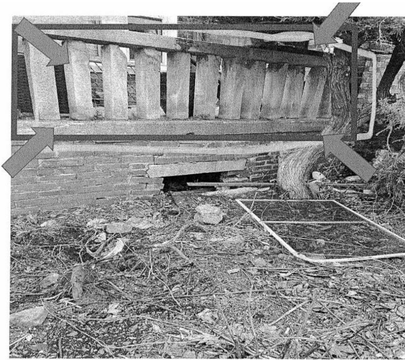
Restoration of Handrail
