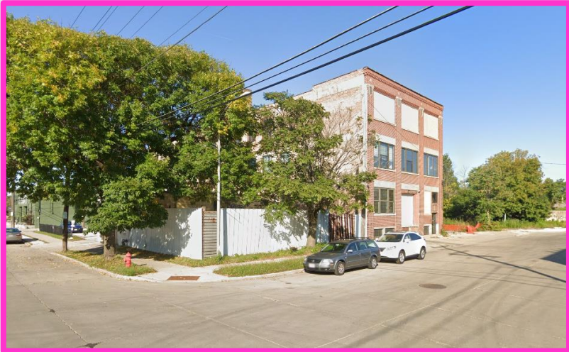
View from E Mineral St looking northeast
