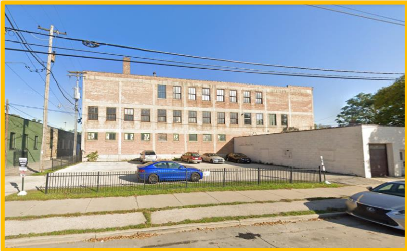
View from S Barclay St looking east
