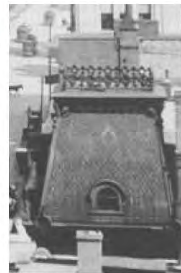
Mansard roof detail.
