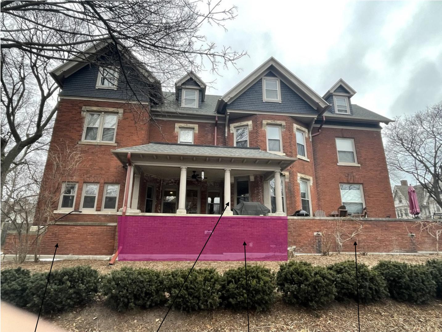
Existing brick masonry porch wall to be reconstructed with matching brick and salvaged stone cap and stone through wall scuppers. Existing stone base will be salvaged and reused or repaired/replaced to match where required.
