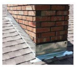
cost. Straight flashing wraps around the base then shingle are installed over top.
