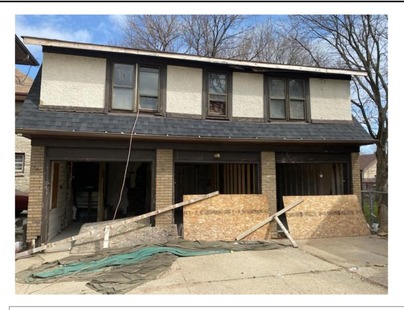
Garage to be repaired including wood trim, wood fascia and wood soffit. At lower left masonry to be repaired.
