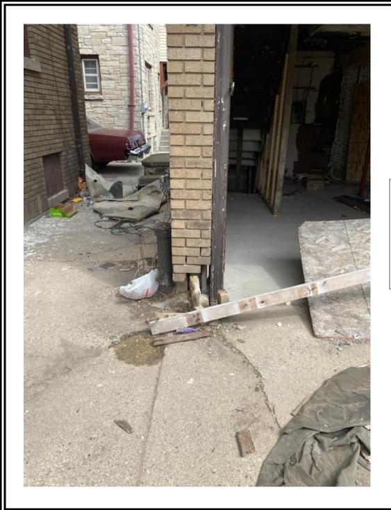
Masonry to be repaired re-using same brick. If additional brick is needed the new brick will match the existing.
